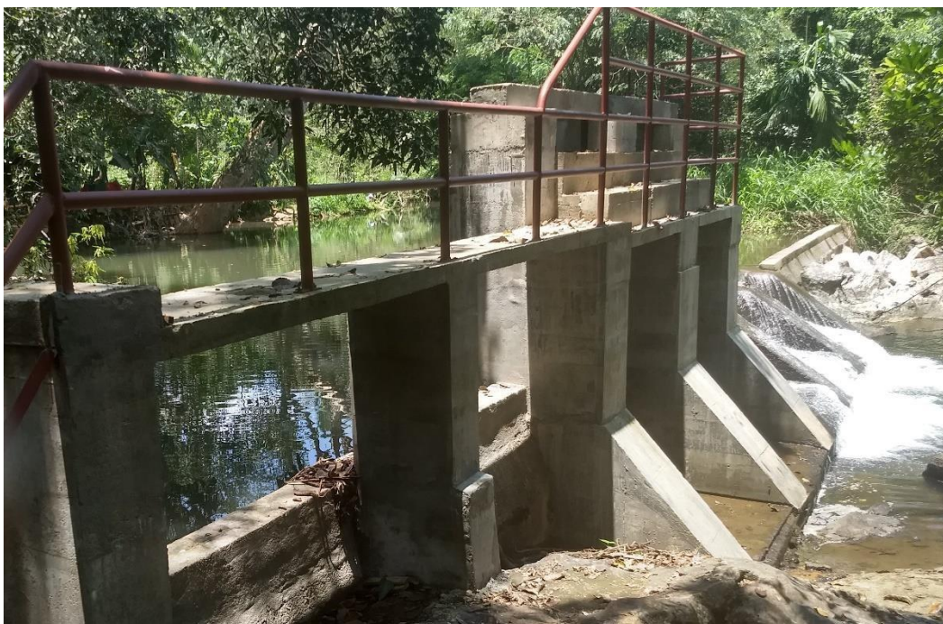
Figure 4: Canal infrastructure rehabilitated by Farmers' Association
